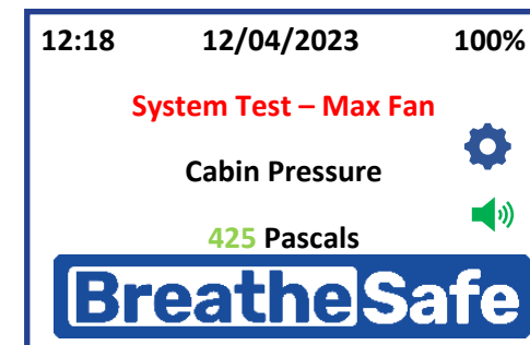
Record / Photograph the cabin pressure result (Max Fan Speed).
